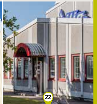
Property Kupolen 3 Address Krossverksg. 7-17 Area 10 037 m 2
